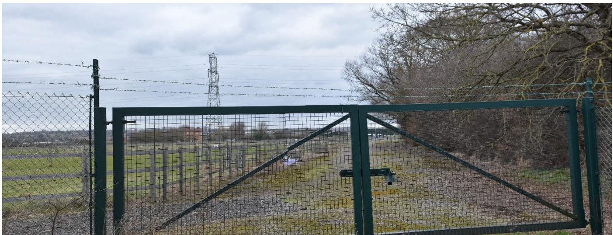
Plate 3. View towards point of connection from Wash Road
